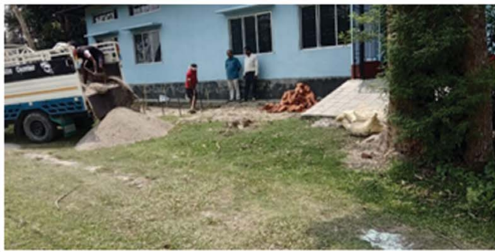
Fig: Construction of CFC underway
