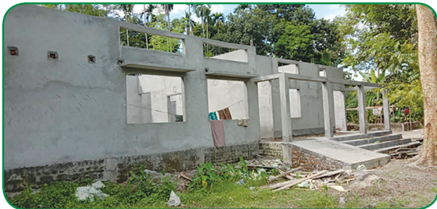
Fig: CFC Building under construction
