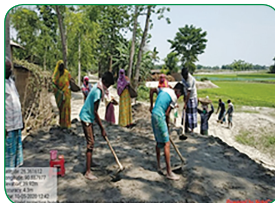
Construction of Agri bund Barpeta
