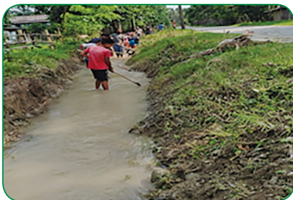
MGNREGA Canal Work in Baksa
